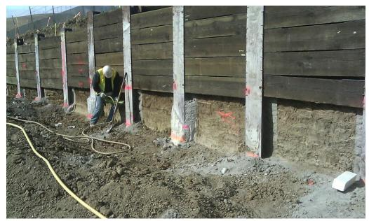
Figure 8.2: Bracing of Timber Lagging
