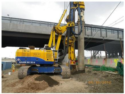
Figure 8.1: Drilling of Steel Casing for Installation of HP Sections
